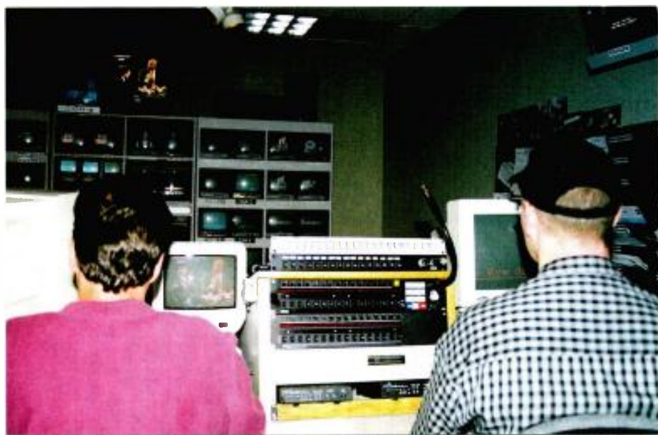
The "B" control producer's station, shown here, provides full communication to both local and remote locations (some 30 miles away) through the new Telex Adam intercom.
