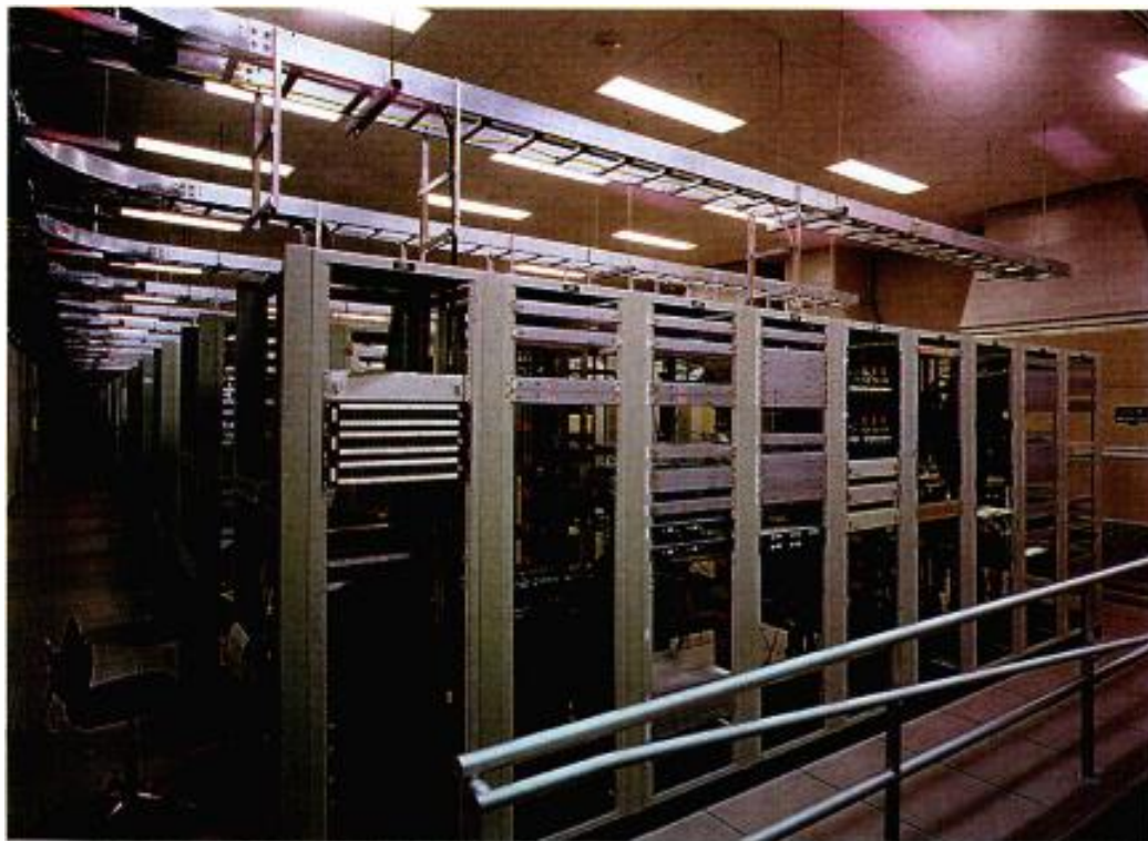
Rack and equipment rooms only get smaller. It's crucial to build them larger than initially needed if there's to be room to grow. WJXX-TV technical room begins with 12 rows of deep racks.
